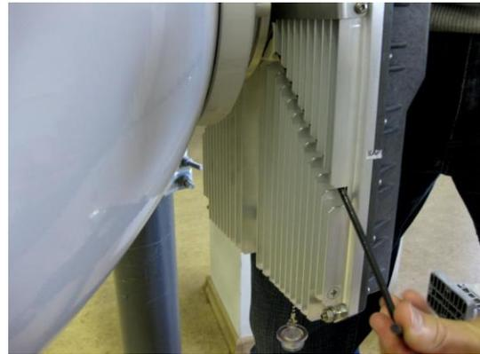
4 Tighten bottom fixation clamps.
